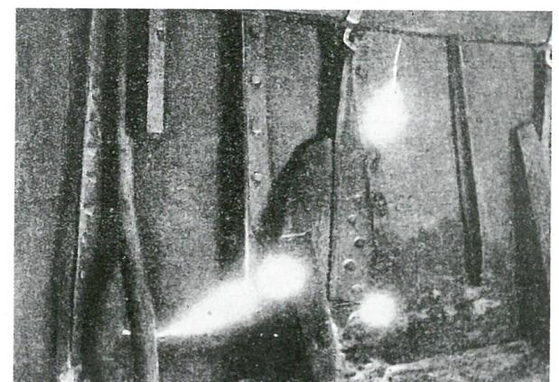
Broken plates in the Chelyuskin's hull. The picture was taken almost in darkness, with chinks of light showing.
